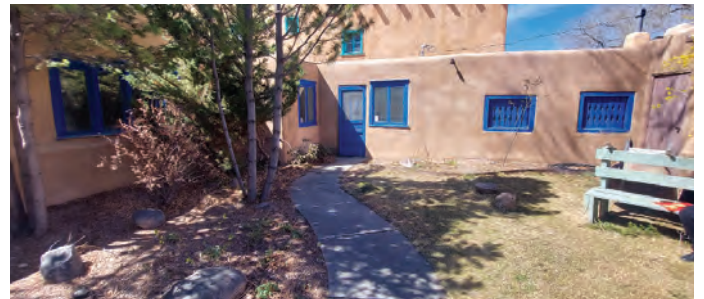
Courtyard 1 looking southwest
